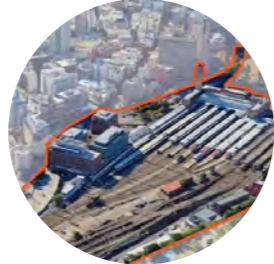
04. Railway Square Redevelopment
