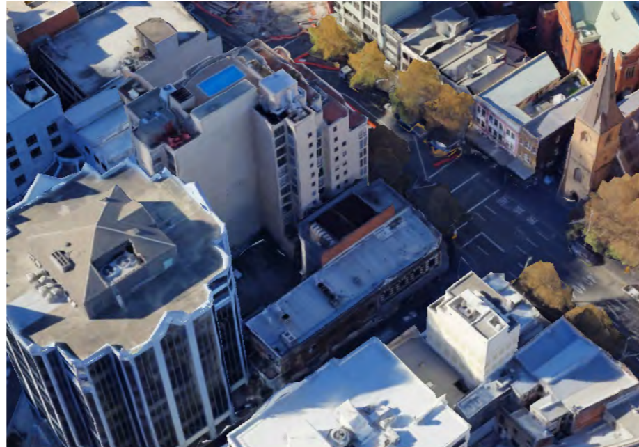
Above: Current Condition, Google Images
