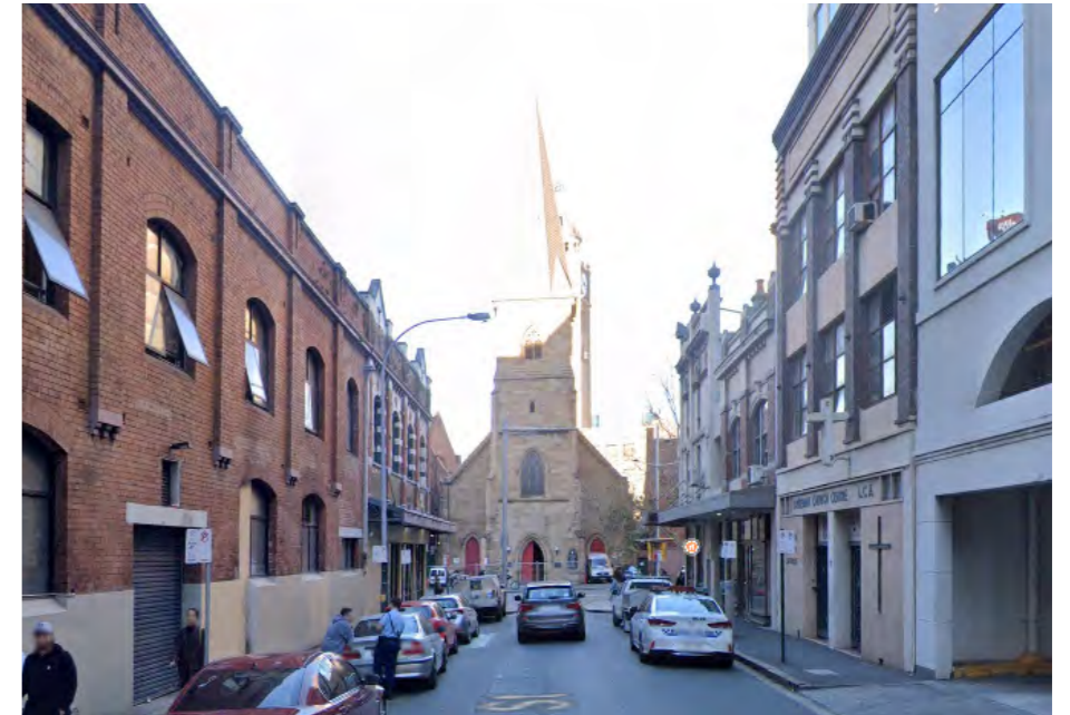
Above: Current Condition, Google Images
