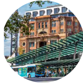
03. Railway Square Bus Terminal
